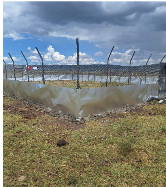
Photos from top: A traditional boma made of sticks and branches. © Dominic Kimani; A predator-proof boma, built with metal supports, fencing and blinds covering the lower portion. © Dominic Kimani
