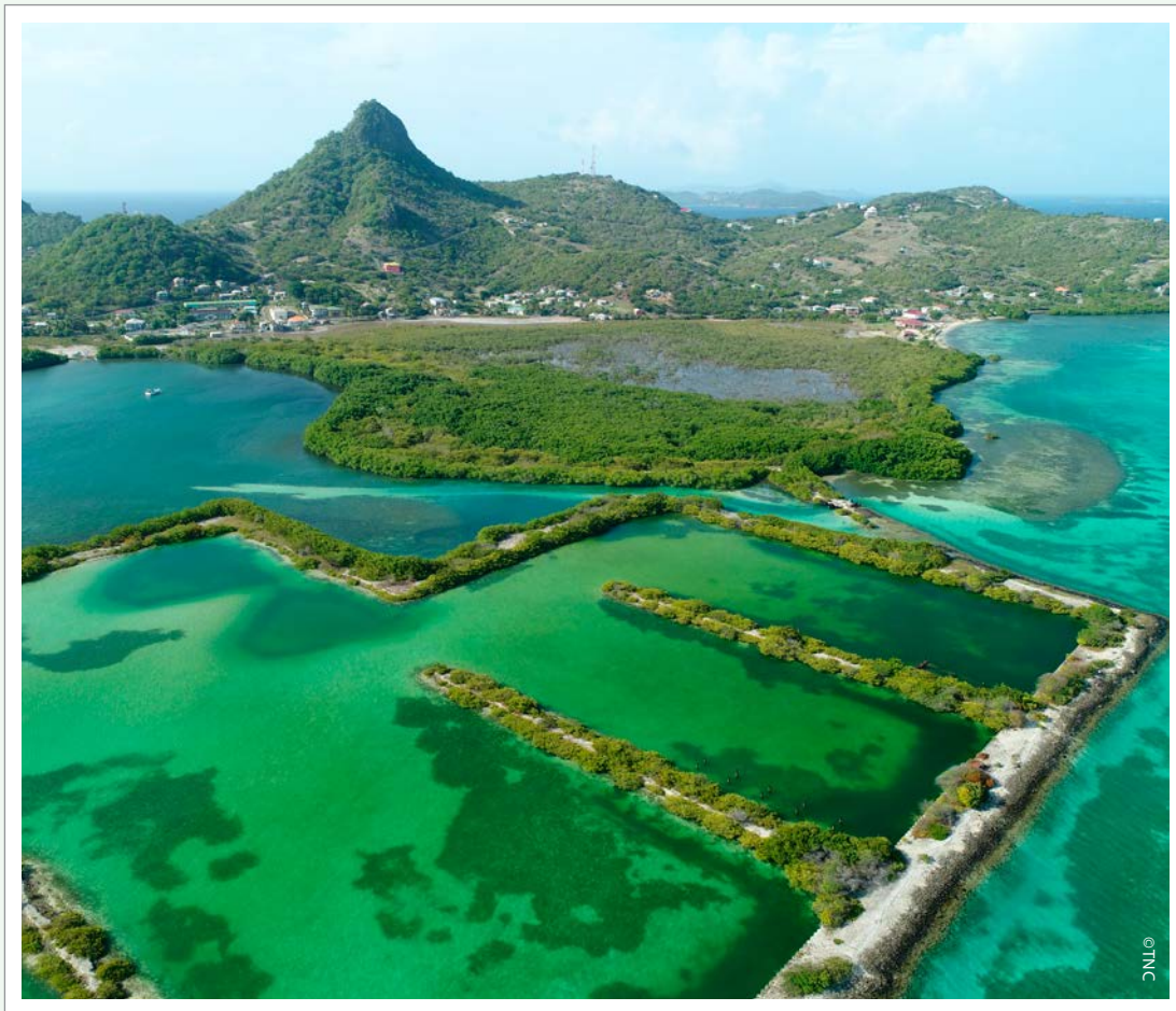
Figure A3.3 Aerial UAS image of Ashton Lagoon, Saint Vincent and the Grenadines taken from a DJI Phantom 4 Pro at an altitude of 120 m on 24 June 2017
