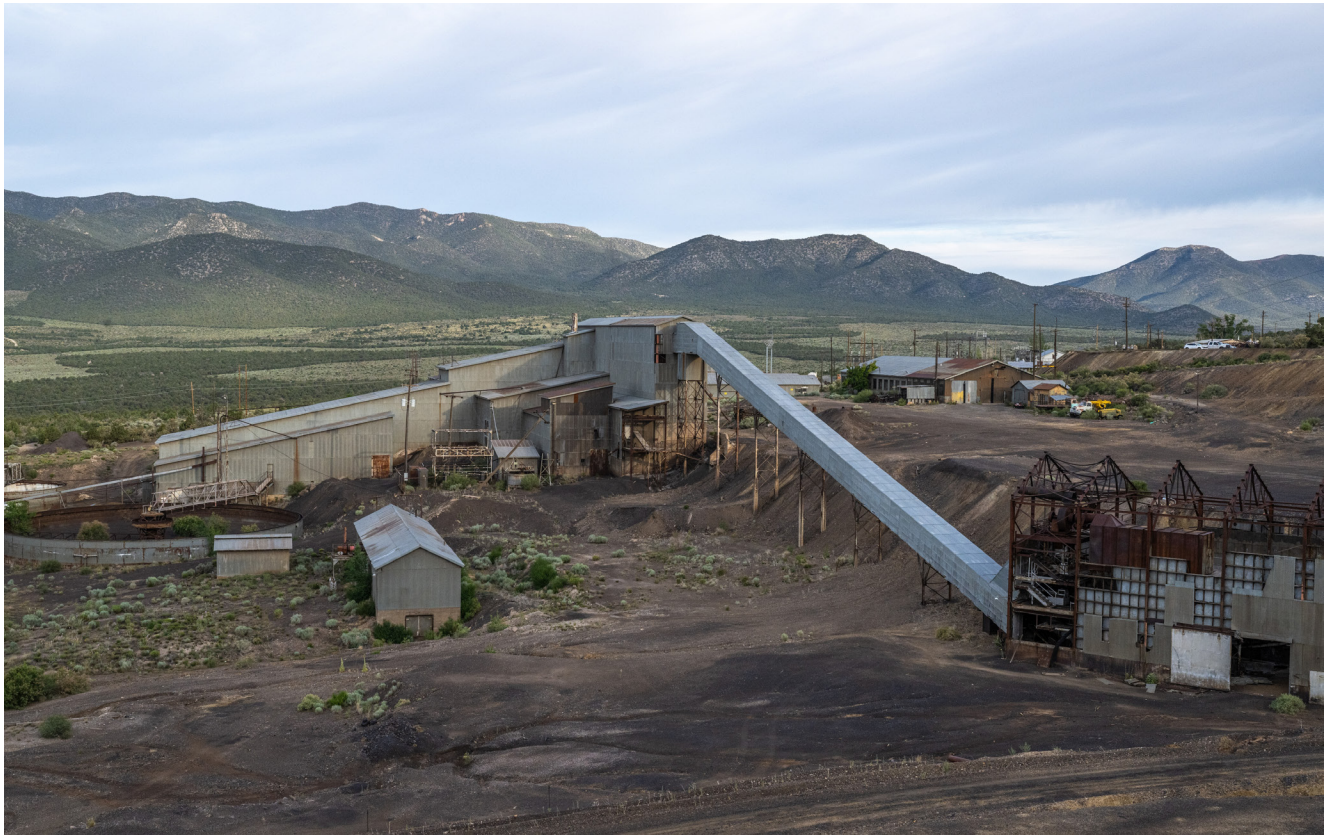
CASELTON MINE AND MILL SITE in Lincoln County near Pioche, Nevada. Caselton is a brownfield site proposed to be used for solar. © Bridget Bennett
