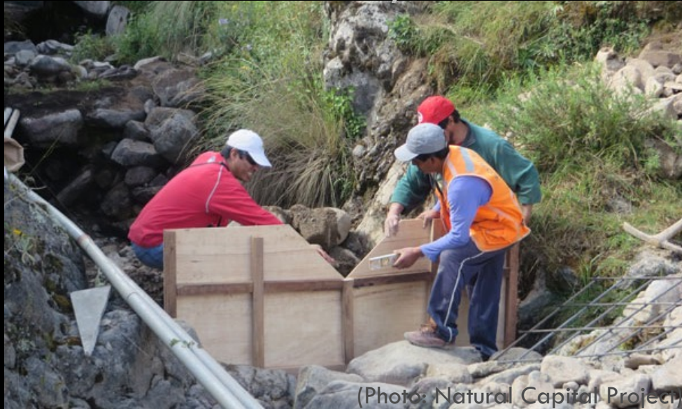
Diversion-Infiltration System Restoration
