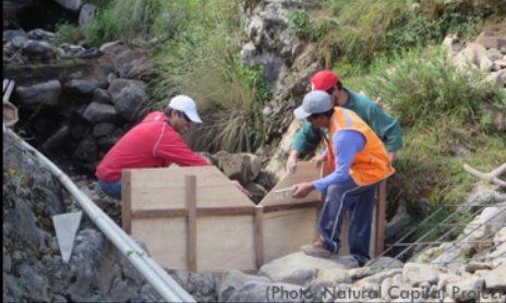
Diversion-Infiltration System Restoration
