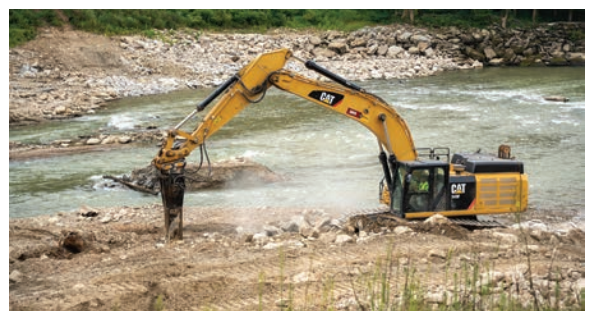
CJ Aquatic Restoration hard at work on dam removal. ©Mike Wilkinson
